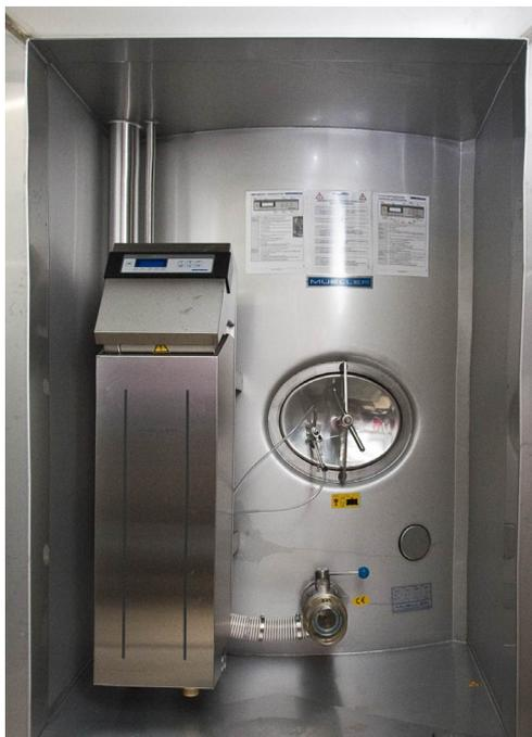
The alcove is the connection between the Silotank and the milking parlour. Through the alcove the manhole, sampling valve, inlet and outlet should be accessible
